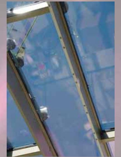
The artificial lighting is integrated discreetly into the glass roof structure. LEDs make this solution possible.
