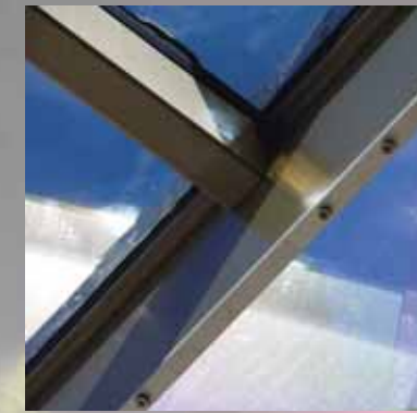
The artificial lighting is integrated discreetly into the glass roof structure. LEDs make this solution possible.
